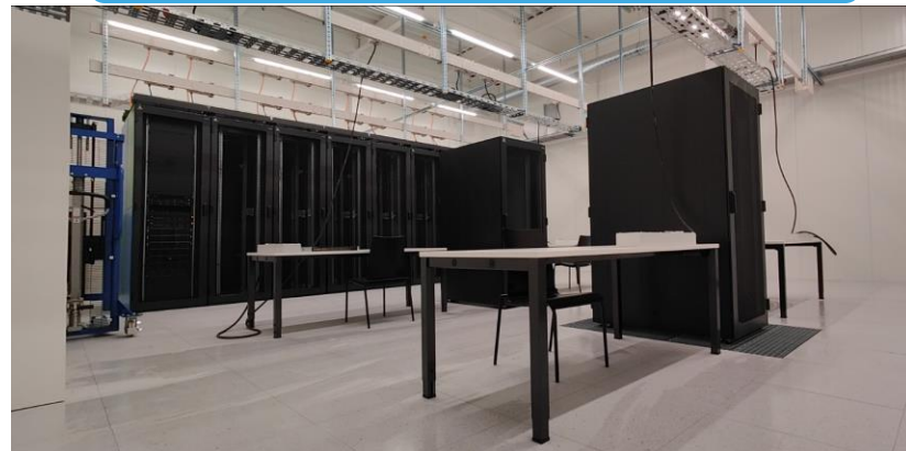
Racks with air/water passive cooling
